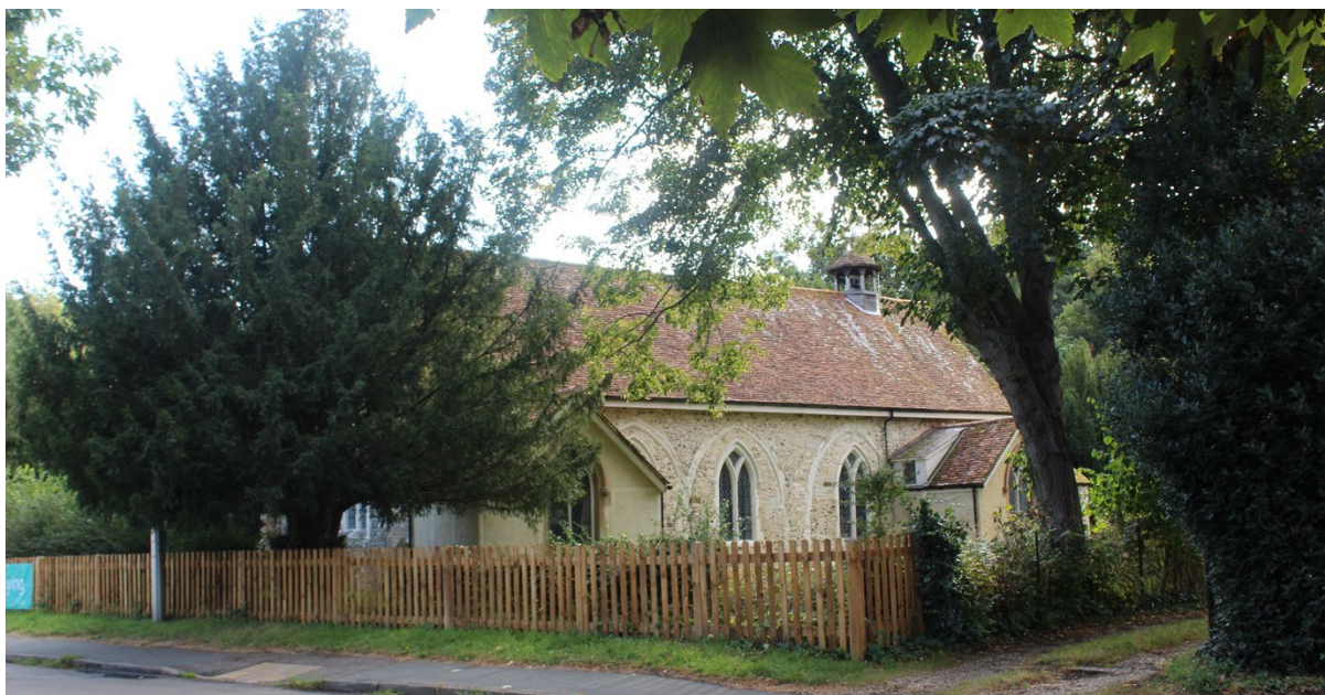
FIGURE 36 VIEW 11 ST MARY'S CHURCH, IN ST MARGARETS PARISH, ON HODDESDON ROAD St Mary's Church in the Parish of St Margarets is a very well-loved landmark. Recently the building has been renovated following enormous efforts to raise money so that it looks very well cared for and historic. The attractive picket fence demarcates the grounds which includes a graveyard and there is a sense of tranquillity and welcome.
