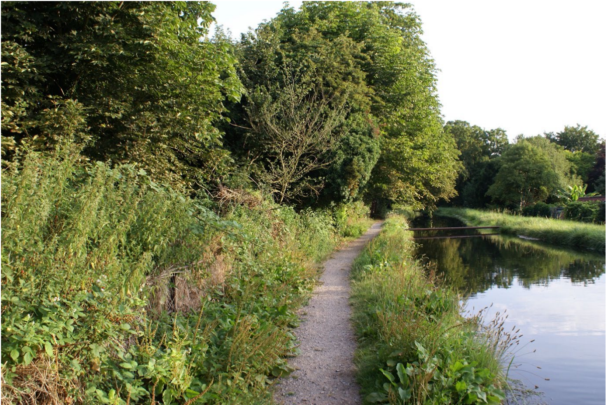
FIGURE 40 LGS3 ST MARGARETSBURY ESTATE BY THE NEW RIVER PATH
